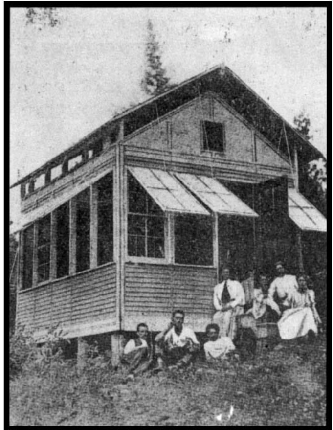
In the summer, many of Yungborn's guests stayed in 'air cabins' which were specially constructed to maximize circulation. Note the special roof construction to allow "healing" fresh air to constantly circulate though the building.
